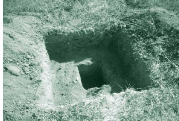
Preparing a pit trench
