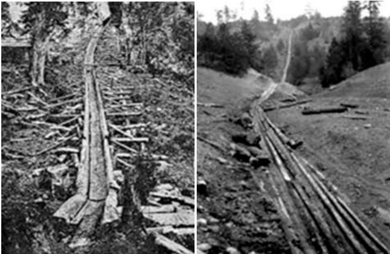
Figure 1. Permanent chutes built from logs (USA early 1900s)
