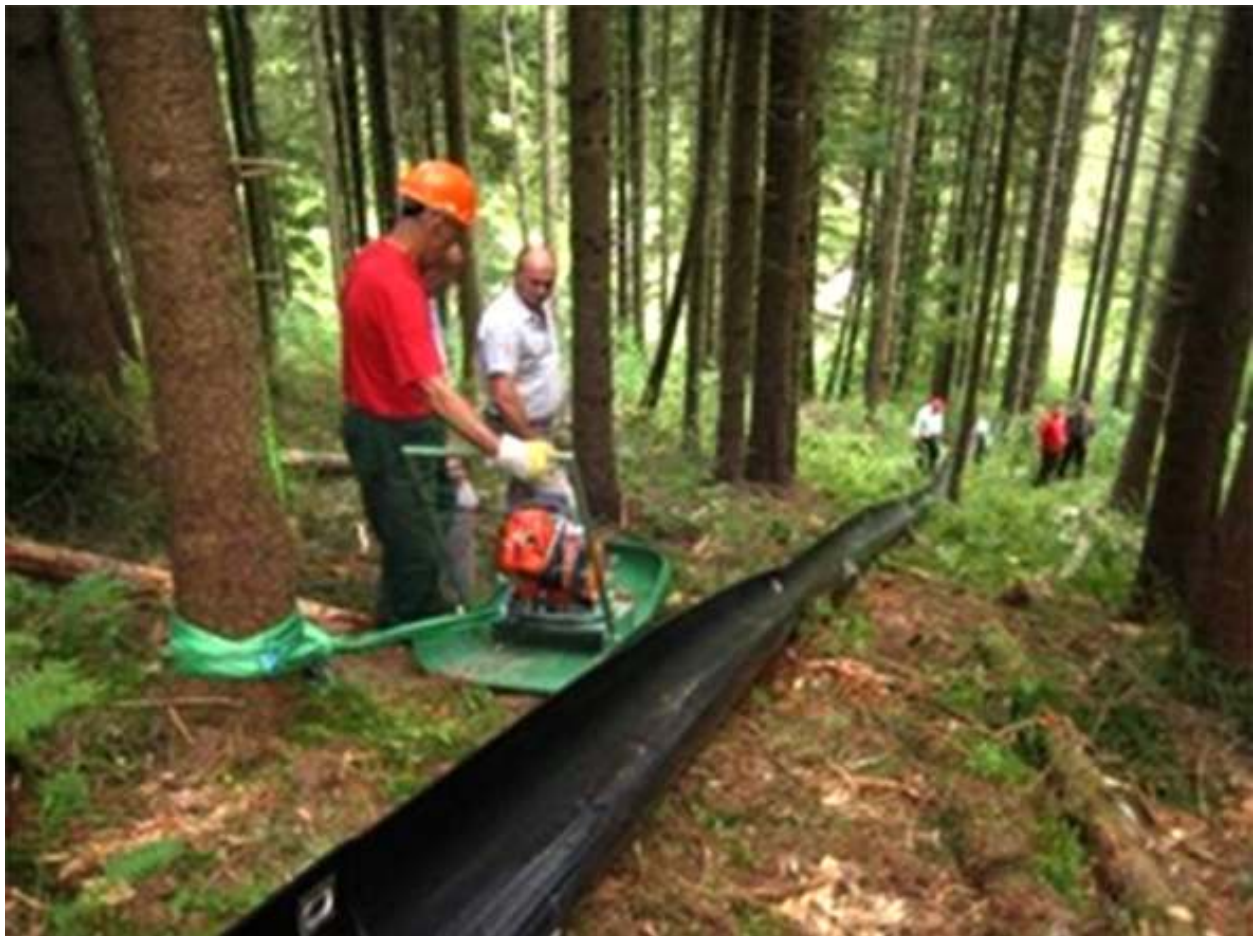
Figure 2. Leykam logline installation with mobile winch (Acar 2005)
