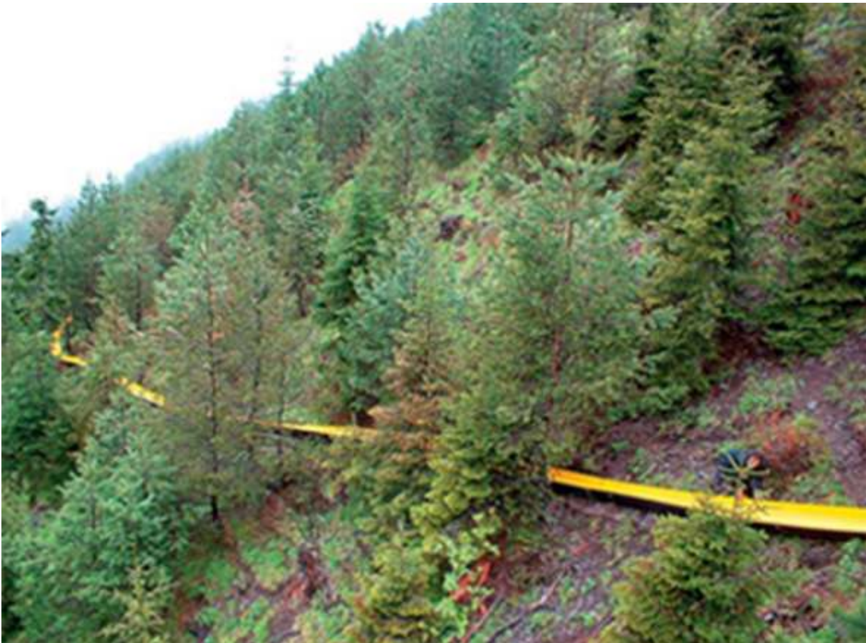
Figure 8. Set-up of 260 m extraction line on slope averaging 30 percent
